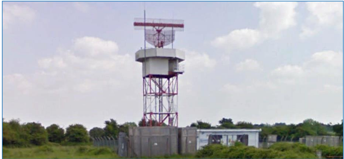
Figure 2: Shannon Airport PSR with co-mounted MSSR
